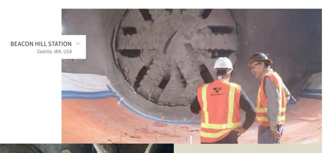
Beacon Hill Station is a deep-mined underground station located in complex glacial soils with multiple groundwater horizons. DSP was retained as a specialist consultant for the final design of the large NATM / SEM / SCL station tunnels, as well as various cross passages and adits.
