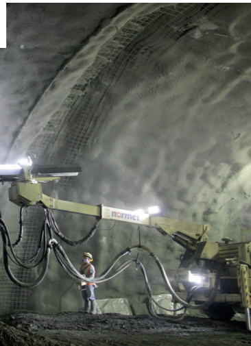
SPRAYED CONCRETE for ground support
