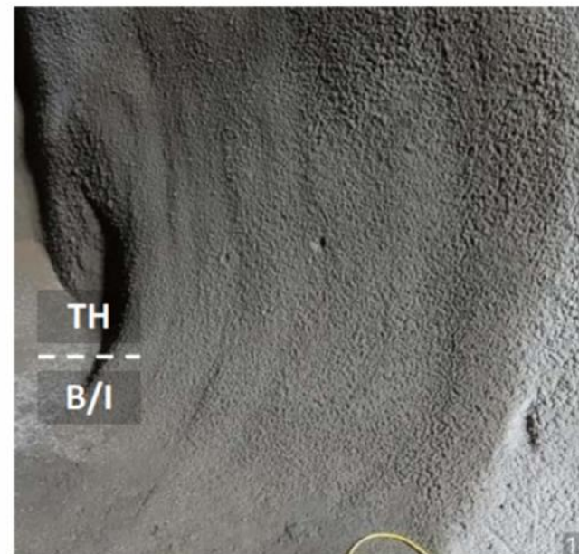
Step 3: Primary lining to full thickness
