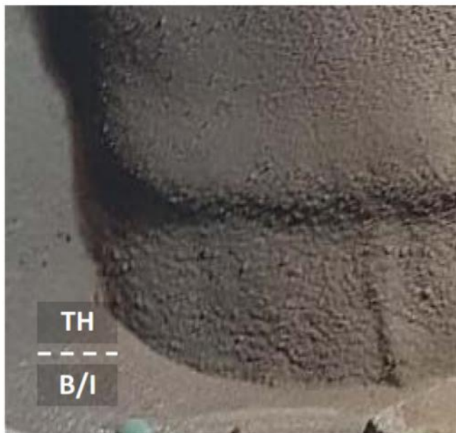
Step 1: Primary SCL at stepped joint
