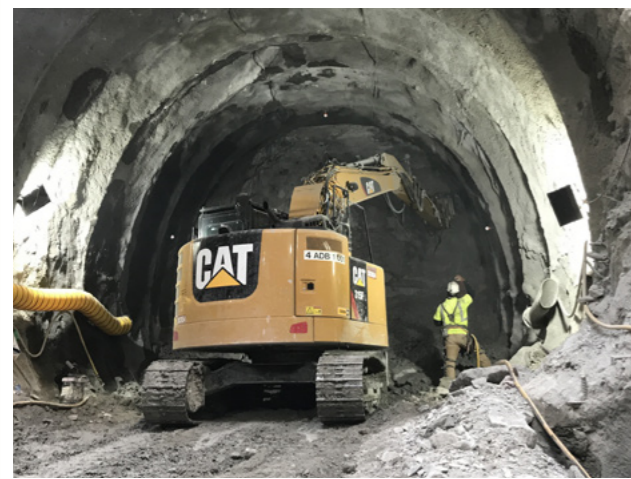
^ TBM Starter Tunnel
